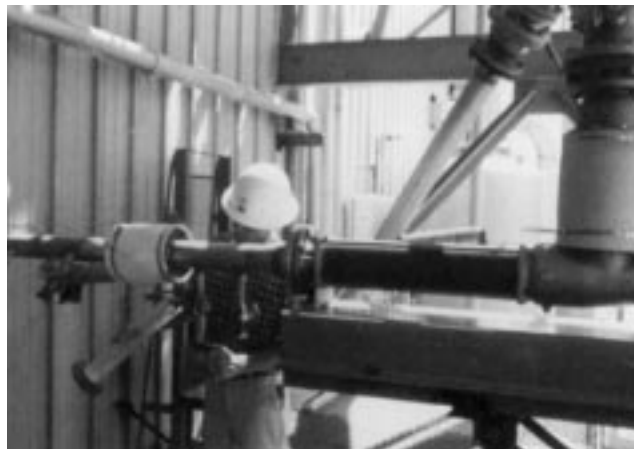
Photo 1. This progressive cavity pump is one of three transferring boric acid crystals from cone/settler tanks to a vacuum belt for additional dewatering at Borax's Boron, CA facility.
